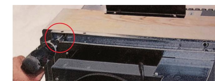
30 Prepare the condensation water hose connection on the base of the conditioner unit by removing the plastic shroud over the hose connector outlet.
