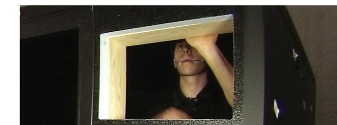
25 Using a pencil, mark the position of the **C1** metal brackets' screw holes on the top and bottom of the timber frame.
