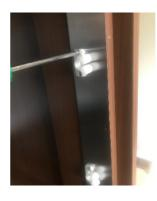
For both sides, align the top and bottom female clips (part 2) with the template screw holes and fix the female clips into place with the 6 gauge screws.
